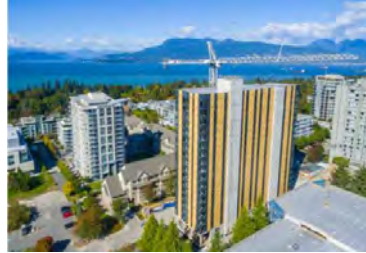
Figure 3: Aerial view of the UBC Brock Commons (Source: photo by K.K. Law)
