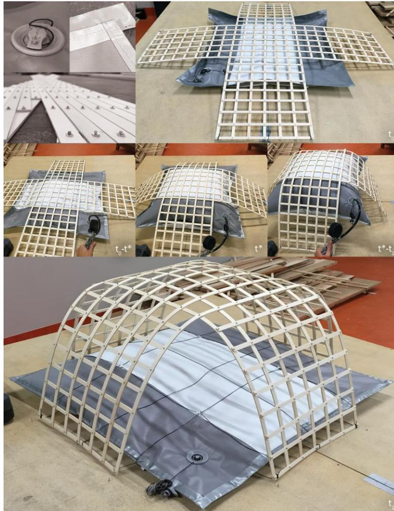
Figure 4: Top left: valve, stitching and joint details. Main: gridshell erection phases from  $t_0$  to  $t_1$ .
