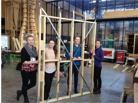
Figure 3: Week 13 – A group of 4 students has constructed a shed wall to AS1684.2-2010
