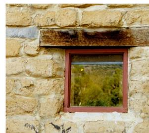
**Figure 11:** Mud brick and timber window frames used in Brambuk
