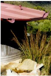
**Figure 15:** Brambuk's design incorporates water spouts which direct the roof's run-off into stone pools beneath them. When it rains the sound of the water falling into the pools is heard along with the rain falling on the roof.
