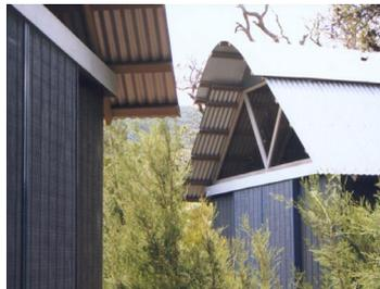
**Figure 10:** Zincalume roofing and *ecoply* used in the Cabins were rated poorly
